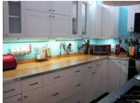
Custom Under Cabinet Installation Cool White 6500K
