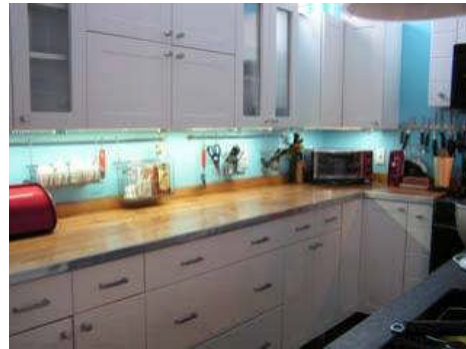
2006 Custom Under Cabinet Installation Cool White 6500K
