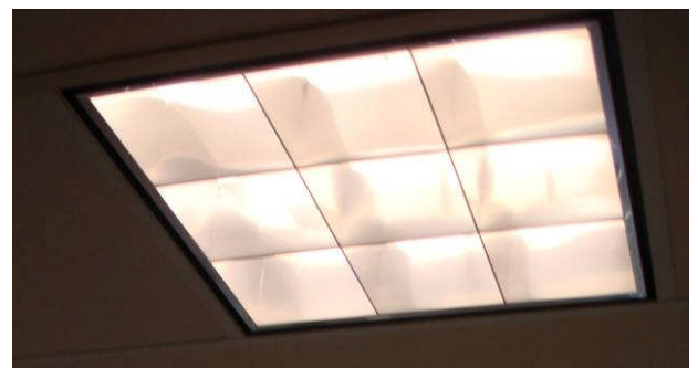
Existing Warm White 27 Foot Candles ~90 Watts
