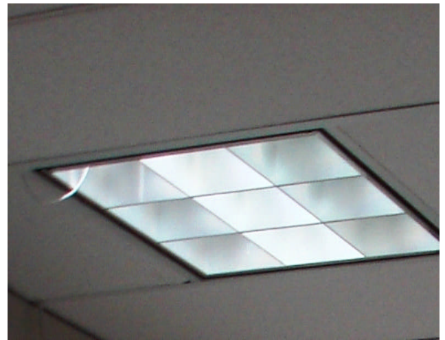
LED Retrofit 57 Foot Candles ~35 Watts
